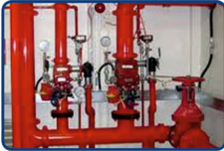
Fire protection system installation work
