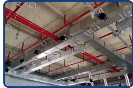
Fire sprinkler system installation work
